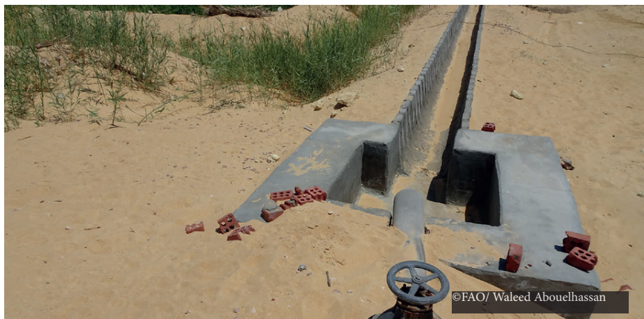
Pumping groundwater into drip irrigation in Siwa.
